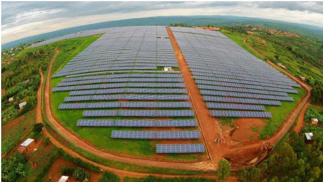
Gigawatt Global launches East Africa’s first utility-scale solar field constructed in the shape of the African continent
